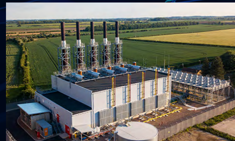
HiIROC 'Gas peaking' plant
