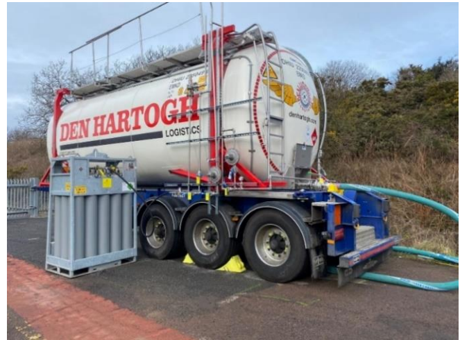
Figure 2 Bio-methanol 30,000L storage tank with nitrogen blanketing system installed at RWG test facility
