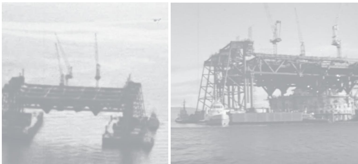
Figure 15 NCP MSF float-over installation on the GBS
